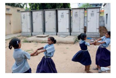
**Climate Impact:** The bioloo disposes human waste in a 100% eco-friendly manner, saves energy and water (no flush toilet) and produces bio-gas. It treats the human waste as a resource that can be re-used, and removes the need for transport of the faeces. It prevents contamination of groundwater with pathogens, and does not require any external infrastructure. The bioloos are a great technical solution for climate mitigation and adaptation.
